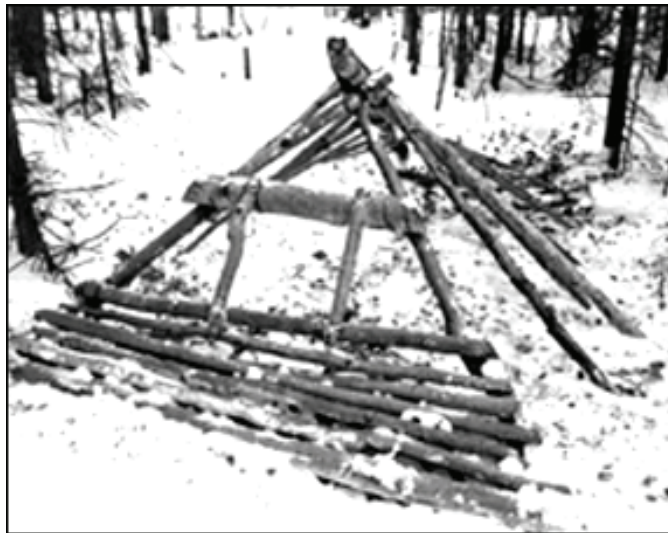
Figure 2-1. Frame of infrared counterdetection (thermal) shelter
