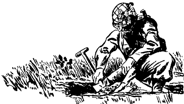
SPOIL BEING REMOVED CORRECTLY
