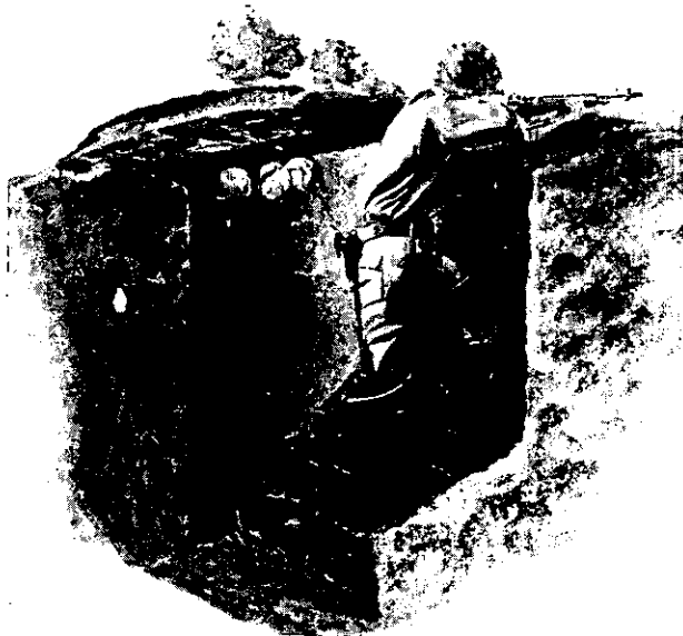
Figure 2-10. One-man foxhole with half-cover.
