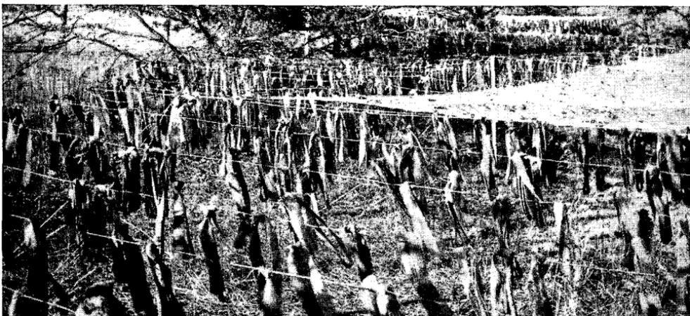
FIGURE 51.—Prefabricated garlands can be used to tie-in a camouflaged installation with nearby natural foliage, or to thicken overhead cover, or to cover spoil and paths. However, light-colored surfaces must be darkened by toning down or texturing before they can be effectively concealed with garlands or garnishing.
