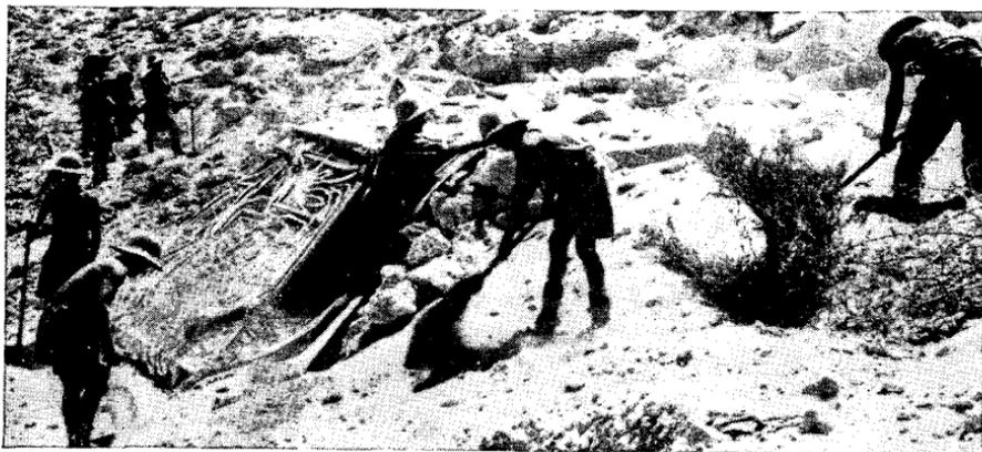
FIGURE 14.—British 25-pounder position located against an escarpment. Use was made of dummy stones in blending position with background.
