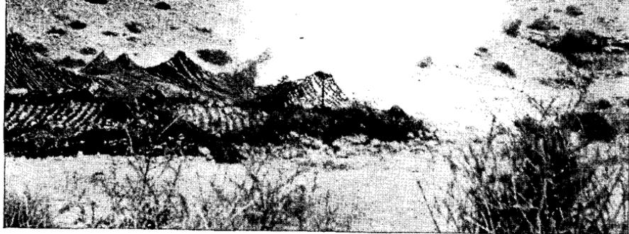
FIGURE 13.—Gun in action. Except for embrasure, camouflage remains in place. Embrasures can be closed quickly after fire mission is complete, or, if piece is moved, drape can be removed quickly.
