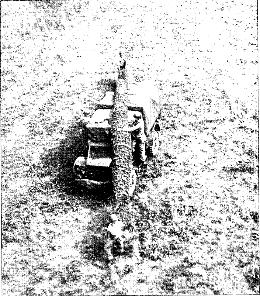
Figure 216. Drape net unfolded diagonally over vehicle.
