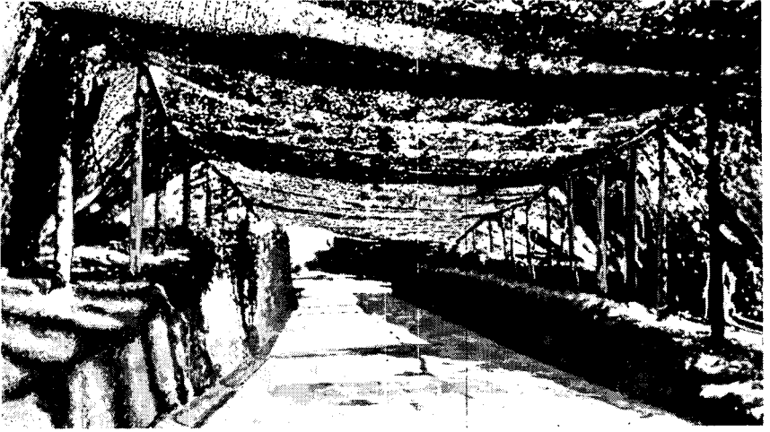
Figure 58. Short access road through cut effectively screened.
