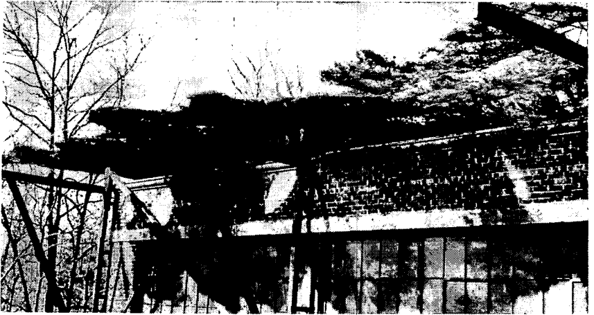
Figure 44. Shape of building distorted through use of garnished netting.
