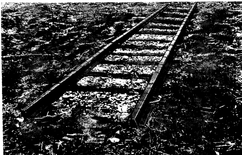
Figure 63. Ties and rails made from flattened and shaped tin.
