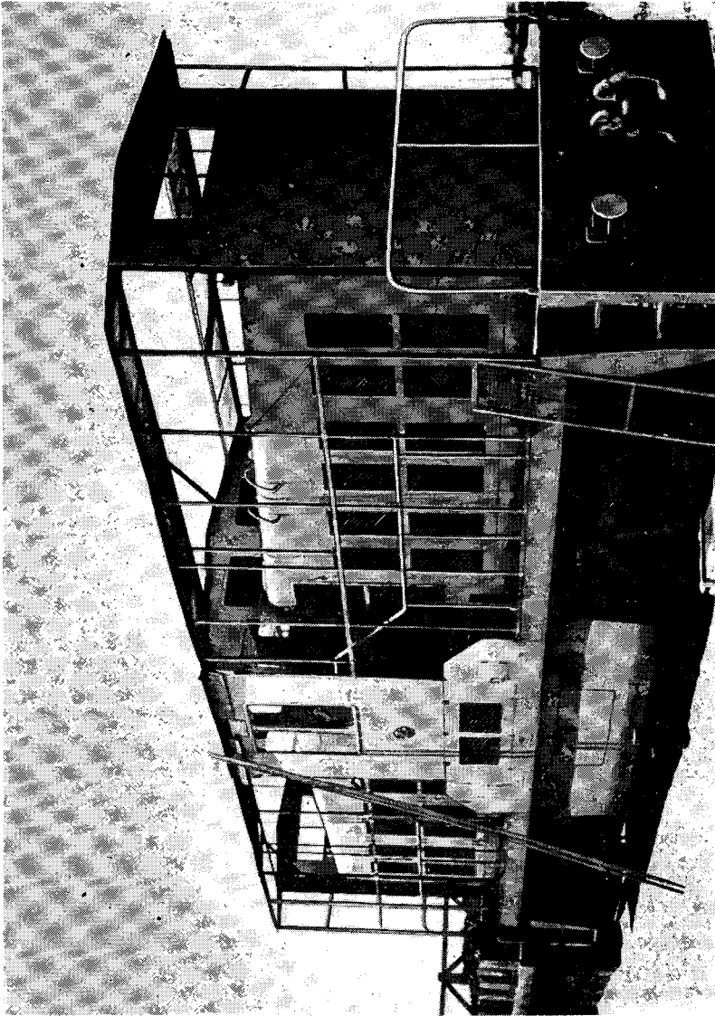
Figure 67. Framework used in disguising Diesel locomotive to resemble bozcar.
