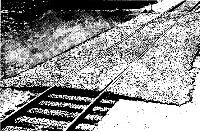
Figure 64. Fitted garnished netting used to conceal ties and ballast.
