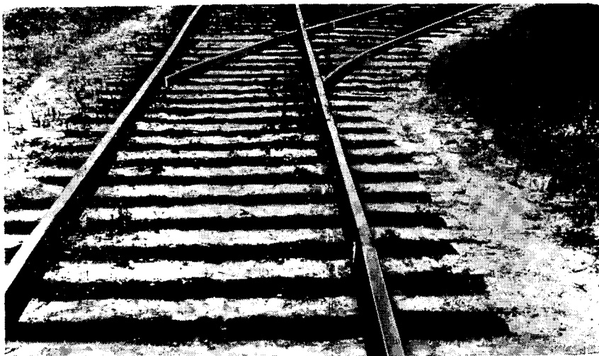
Figure 62. Rails simulated by 2- x 4-inch lumber coated with aluminum paint.
