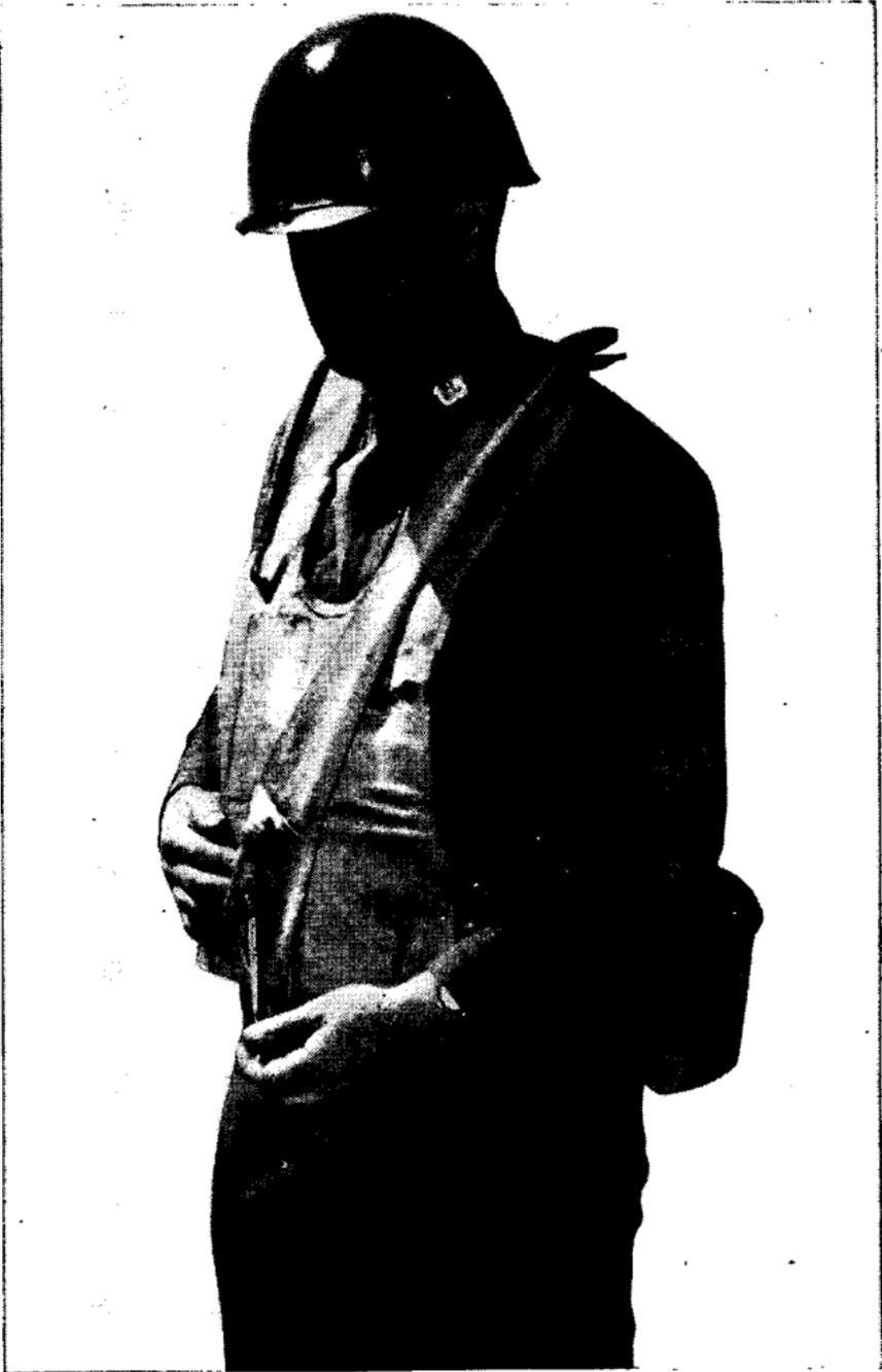
*Figure 7. Inflation-type life jacket being inflated by cartridge.*
