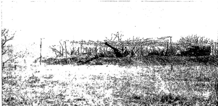
FIGURE 53.—This photograph illustrates a dug-in 155-mm gun position at which flat-top does not cover all the spoil. Supplementary camouflage is necessary to conceal such a position. Flat-top is extended around edges, either with additional nets or with garlands.
